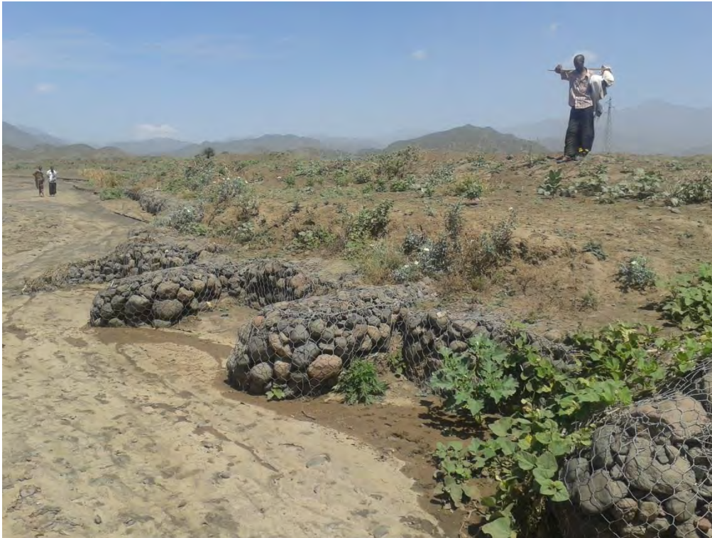
Figure 4.12 - Installation of gabions
